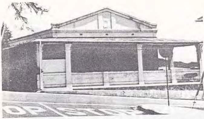
Fig. 24 Directorate of Building Services, Additions to the House of the Deputy Troop Commander, Windhoek, 1902. (Photograph 1978)
