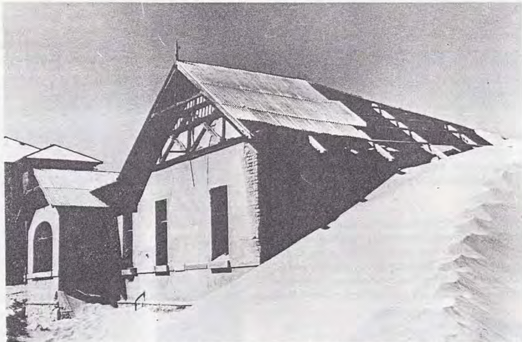
Fig. 39 Remains of a house at Kolmanskop. (Photograph 1979)
